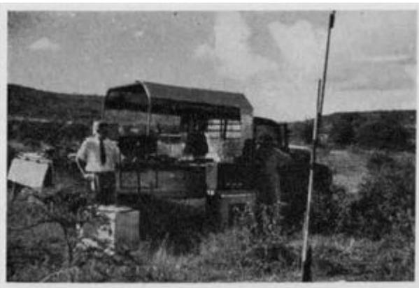
Bechuanaland Geological Survey 3. Bellairs-Enslin electromagnetic apparatus near Lobatsi. Dr. S. H. Shaw from colour transparencies. Plate X.
