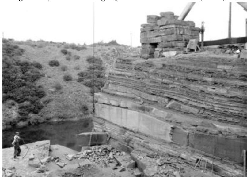
Corsehill Quarry, Annan. Dumfriesshire. New section of quarry. Just after a blast loosened blocks are being raised to surface using a chain sling. Note the differential weathering, the hard sandstones stand proud while the interbedded fine-grained silty mudstones being softer, are
