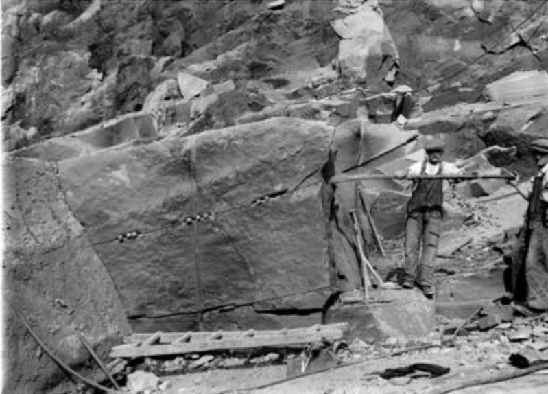
Locharbriggs Quarry, Dumfriesshire. A close-up showing the 'shot-grove' and chisel wedge method of splitting stone. Widely spaced holes are drilled and filled with black powder; once blown and the blocks dislodged, chisel wedges are driven in along planes of weakness (usually bedding planes) to further work the stone. Note the quarryman wielding the large crowbar. The Locharbriggs Sandstone Formation is of Permian age.
