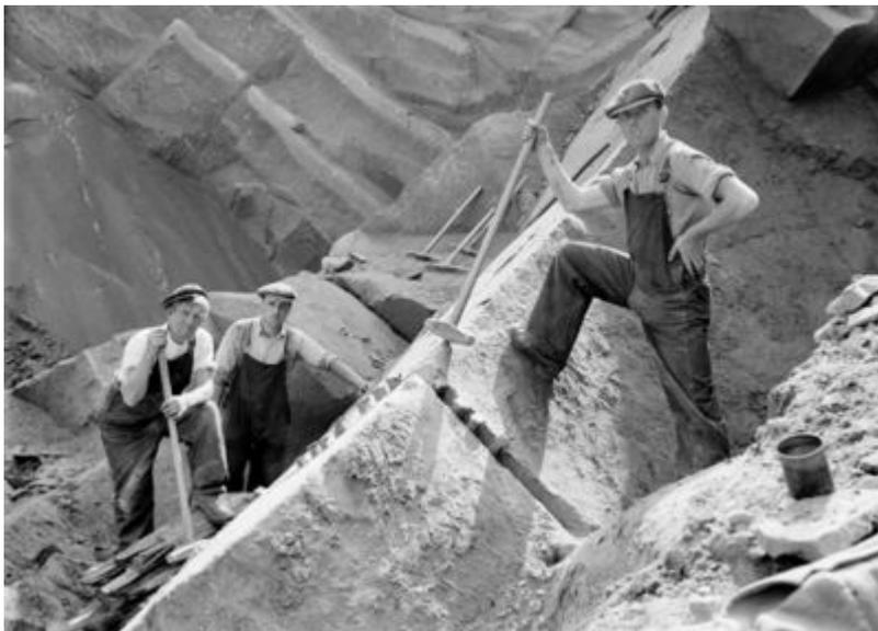
Corncockle Quarry, Lochmaben. The close up shows use of the chisel wedge method to split the stone to the required dimensions. BGS Photograph C3606, P000100. (1937).
