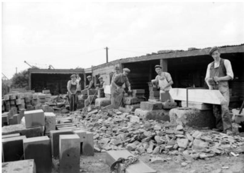
Corsehill Quarry, Annan. In the dressing yard masons are shown at work using mells (wooden mallets) and chisels on the stone. Note that many of the blocks were sawn and that the small holes cut in the faces were used for gripping the block with dogs and chain sling (see block in the foreground). BGS Photograph C3603. P000097 (1937).
