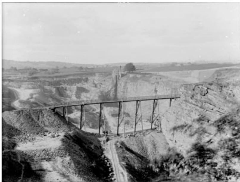
Hailes Quarry, Slateford, Edinburgh. General view of the quarry looking north, with the tramway bridge (not shown on the Ordnance Survey 25 inch County map, 1914 edition) and steam pumping engine in middle distance.
