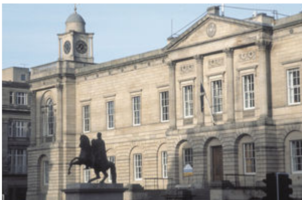
Register House, Edinburgh. Built from
