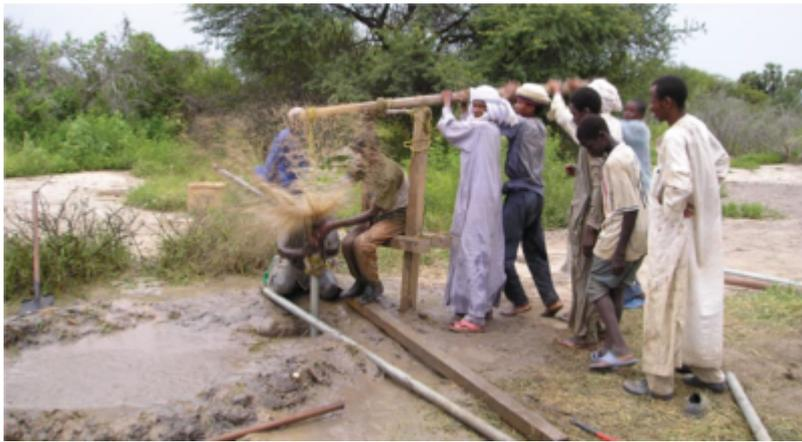
A manual drilling operation in Chad, using the sludging method. Image credit: [PRACTICA Foundation 2009](#)
