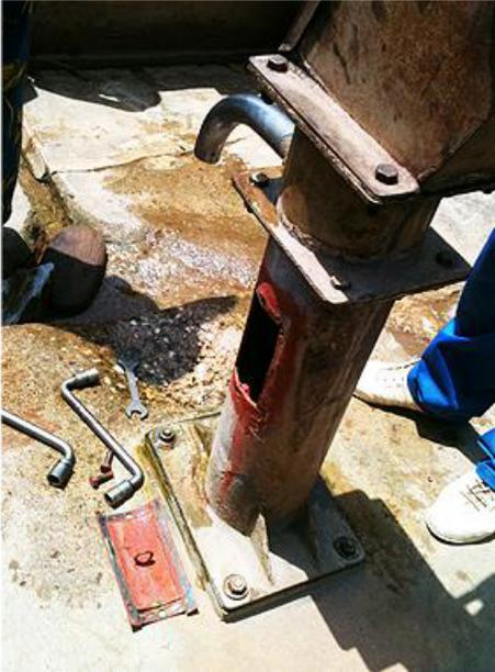
Adapting an India Mark II handpump so that a water level logger can be fitted. Image credit: Richard Carter / WaterAid (2013)
