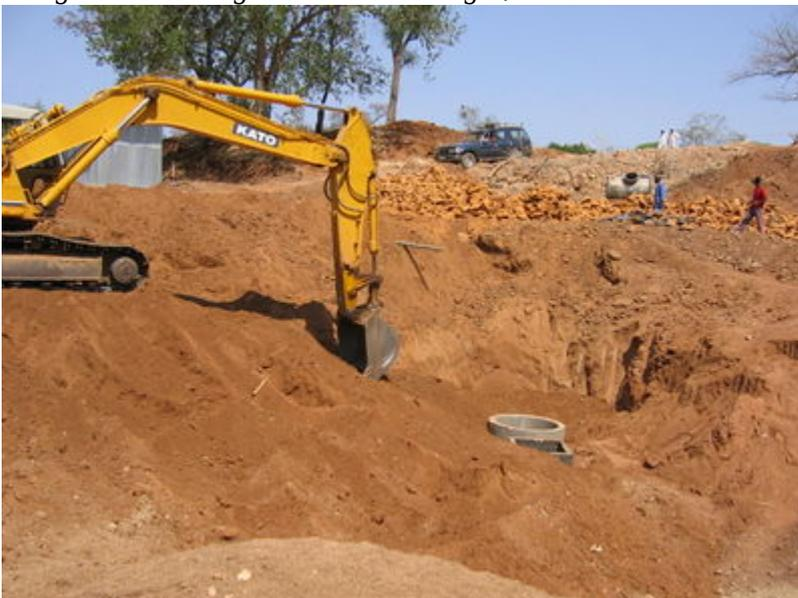
Concrete rings in the alluvial sand aquifer being used to construct a well for groundwater abstraction. Image credit: Brighid Ó Dochartaigh / BGS
