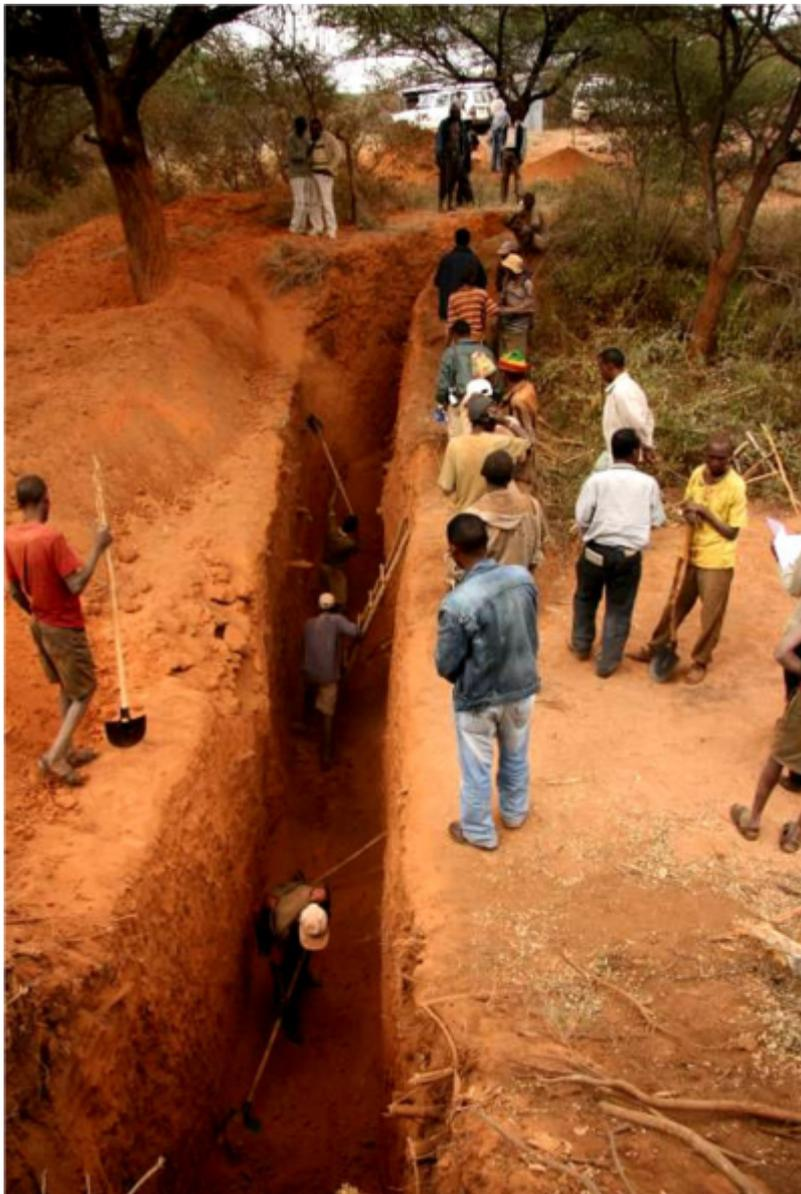
Constructing a groundwater dam in a sand aquifer. An impermeable wall will be built in this trench, preventing
