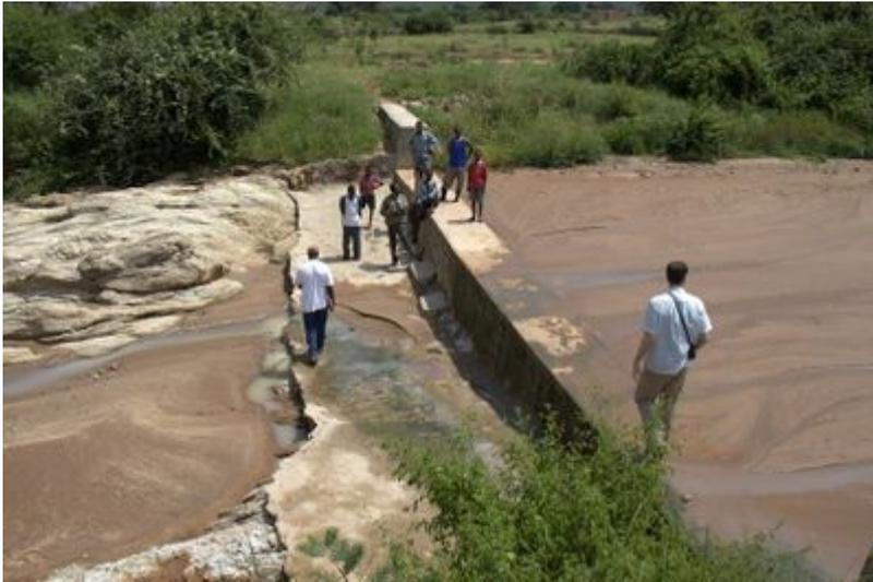
A constructed sand dam in Tanzania. Here we can see only the top of the concrete dam, which extends below the surface. Image credit: [The Mennonite Central Committee Sand Dam Project, Dodoma, Tanzania \(2012\)](#)
