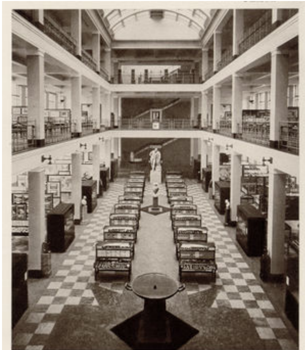
NEW MUSEUM, SOUTH KENSINGTON: Interior View
