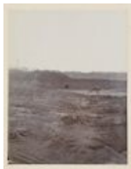
Sections in low level gravels near Ponders End Station.
