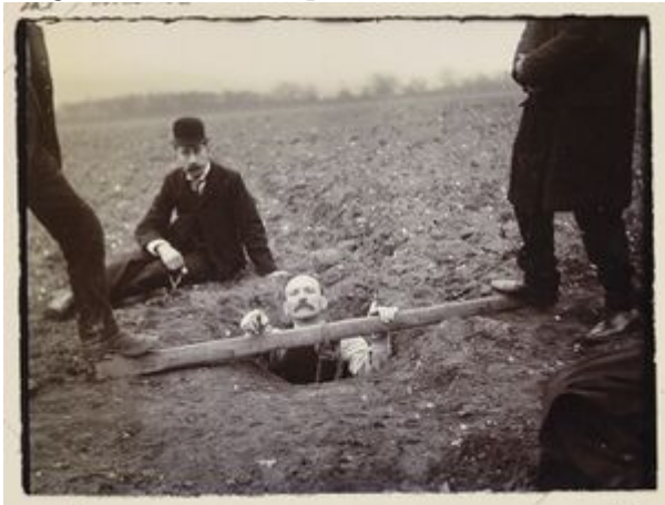
The entrance to a denehole at West Thurrock. Excursion to the Deneholes, Stone, near Dartford. Saturday, February 29th, 1908
