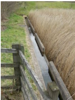
Mine water from Taff Merthyr after treatment emerging from the reed bed treatment area. P802435.
