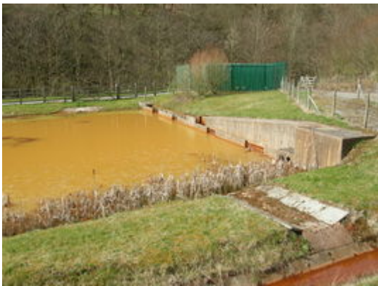
Ferruginous mine water discharged from Taff Merthyr Colliery shaft after closure. P802436.
