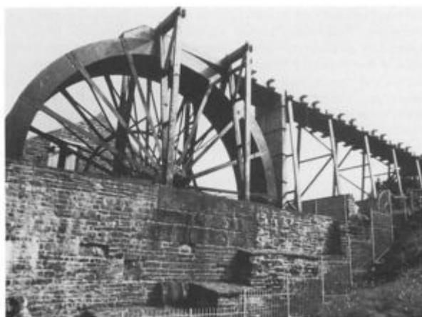
Figure 14.2 Restored overshot wheel, Killhope Lead Mining Centre, Weardale.
